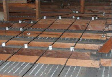
Knob and tube wiring was the first standardized method of electrical wiring in North America, and it was relatively
