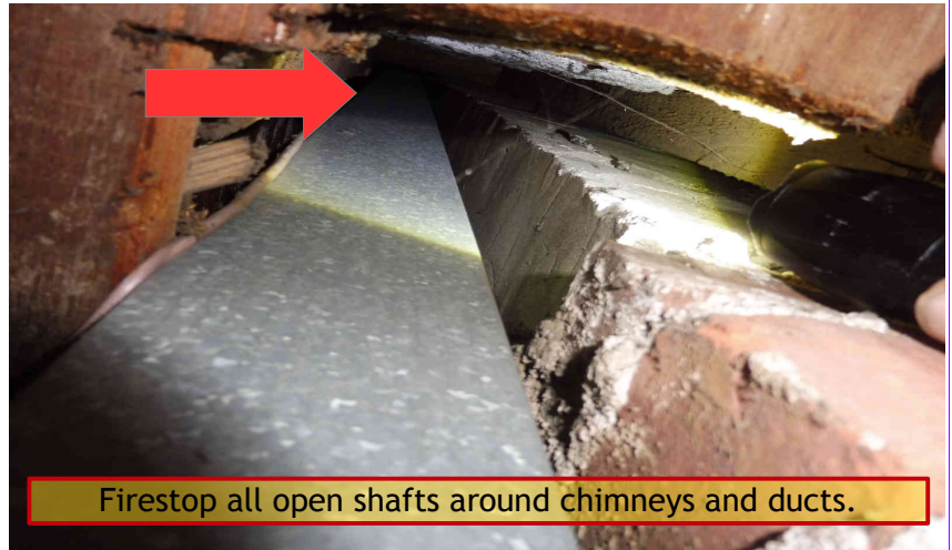
Firestop all open shafts through firewalls (e.g. between buildings, in garages, hallways, etc.)
