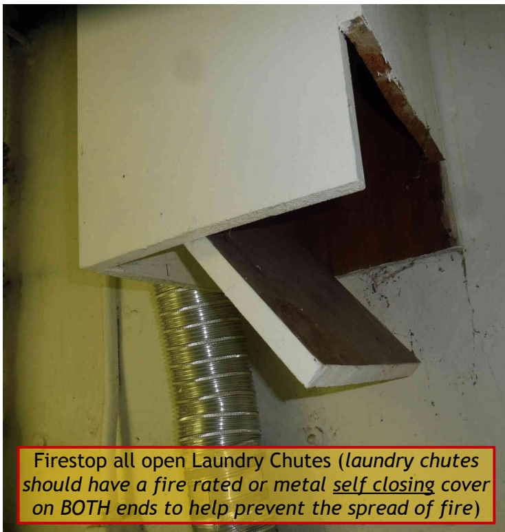
Firestop all open shafts through firewalls (e.g. between buildings, in garages, hallways, etc.)
